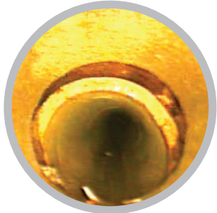
Separated / Offset Pipe
