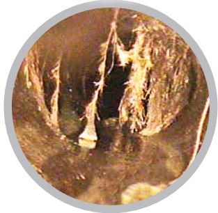
Tree Roots Filling Pipe
