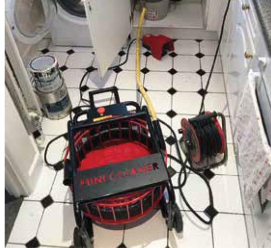
Photo courtesy of MT Drains
